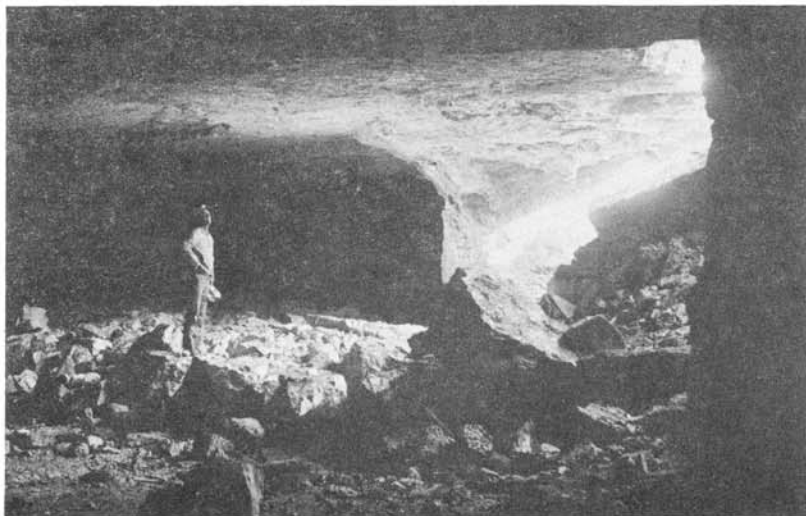
(Top) ROBBING THE ROOF, OR SCALPING , is a common practice where stone removal is the primary concern. However, such practices can only be considered short-sighted, because the removal of a scant two feet of roof rock can mean the difference between a collapsing mine with the mine owner subject to litigation from surface landowners, and a highly profitable operation utilizing mine space with a safe roof. Dotted lines show scalping of about 2 feet of stone. Roof failure occurred within 50 feet of this area (see photo on p. 44 ) (Bottom) ROOF FAILURE has occurred as a result of scalping. Removal of only two feet of stone brought the mine roof dangerously close to the rubble zone at the top of the Bethany Falls, and resulted in collapse of the mine all the way to the surface, creating a large sinkhole and ruining the land for surface development.
